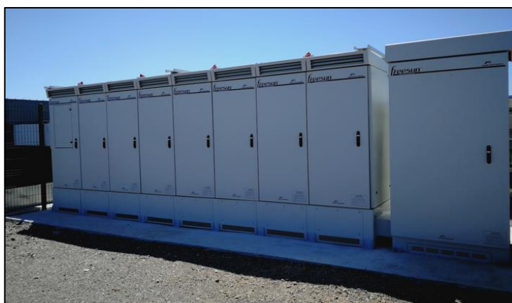
Plate 3-7. Typical outdoor centralised inverter
