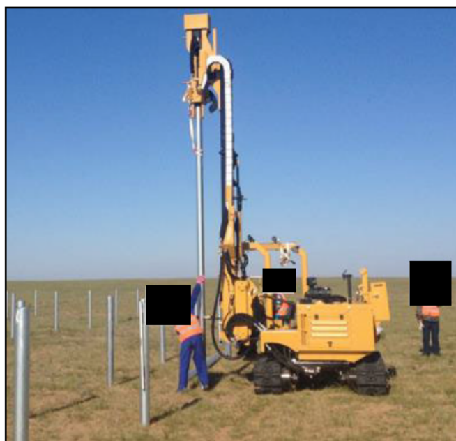
Plate 3-18. Ramming of module mounting structures.
