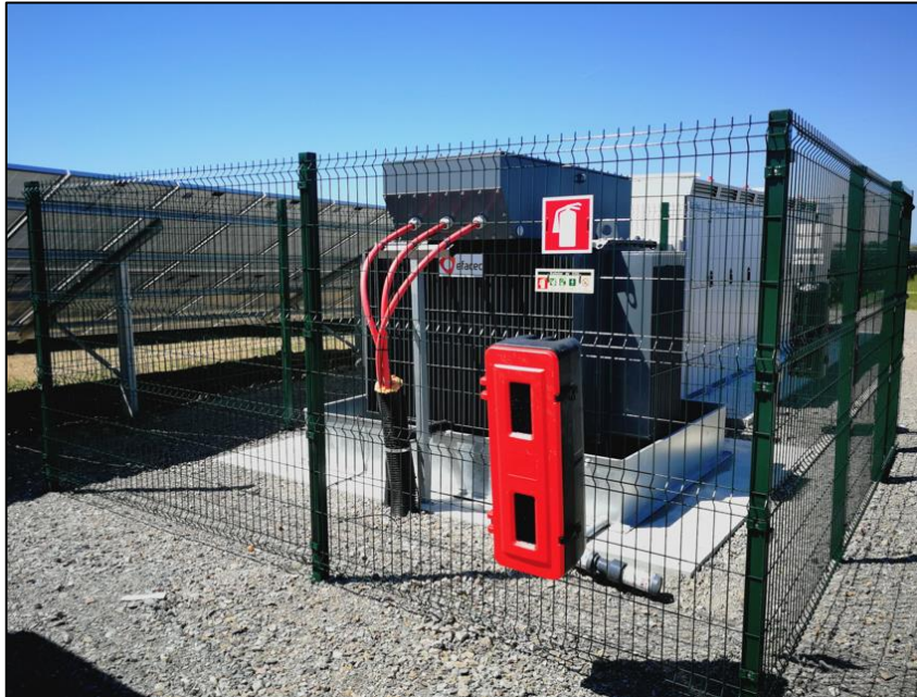
Plate 3-14. Typical transformer compound fencing
