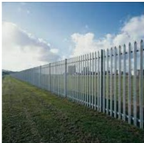
Plate 3-15. Standard palisade fencing
